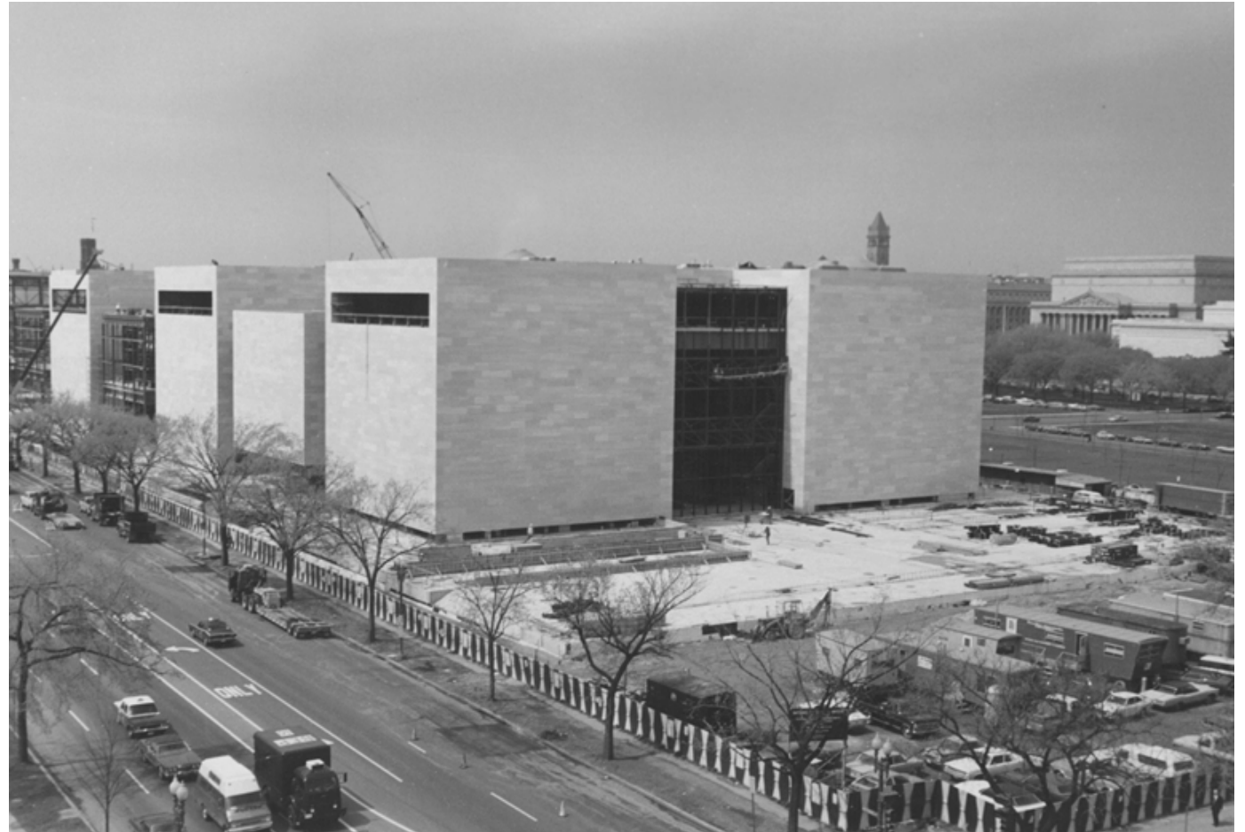
NASM and East Terrace Under Construction, April 30, 1974.
