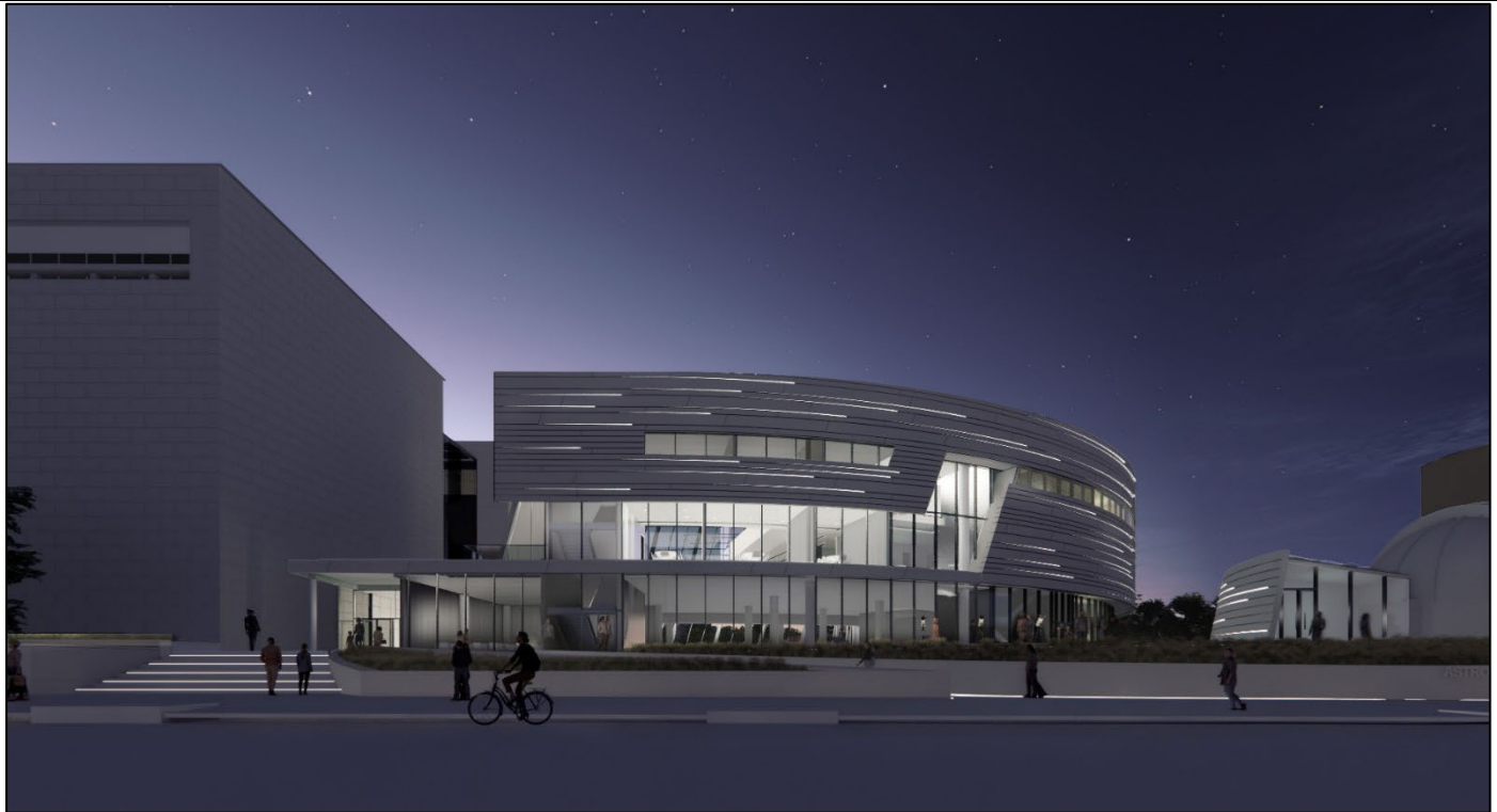
South elevation rendering at night of BLC and Hass Observatory with the integrated façade lighting within the metal panels. (Perkins&Will, 2024)
