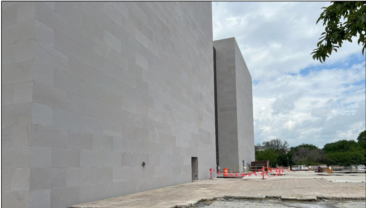
Southeast corner where the new connection will be made with the newly installed Colonial Rose Granite panels. (EHT Traceries, 2024)
