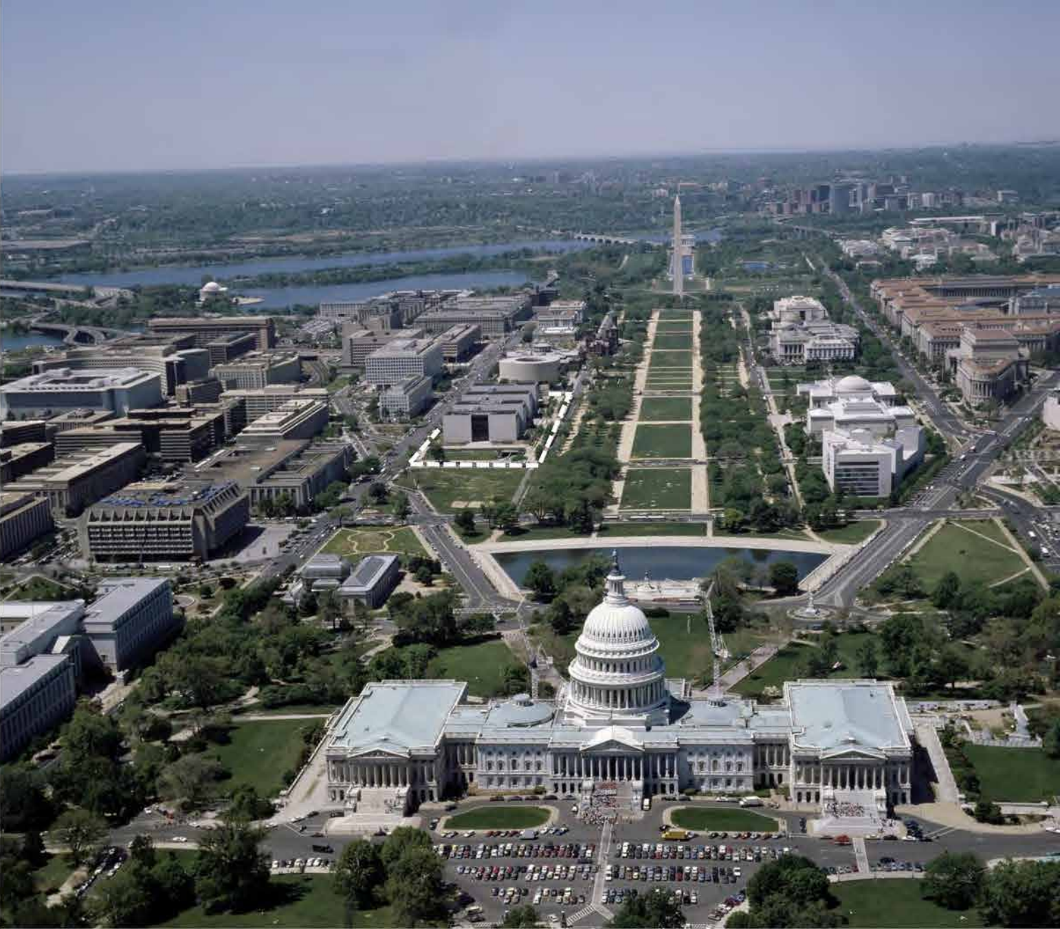
Construct Integrated Bezos Learning Center
