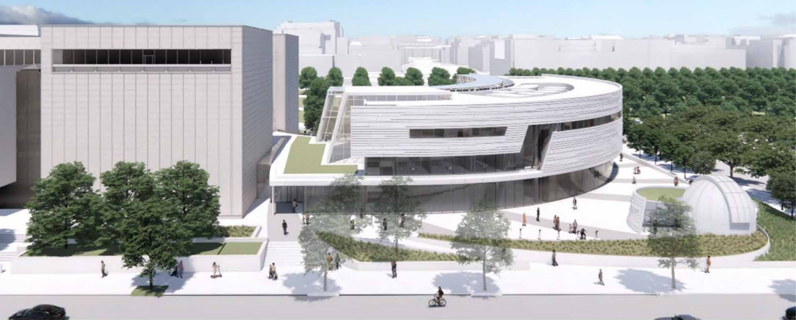
Construct Integrated Bezos Learning Center
