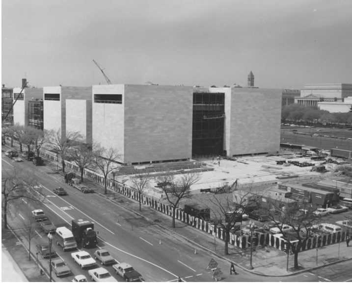
NASM and East Terrace Under Construction, April 30, 1974.
