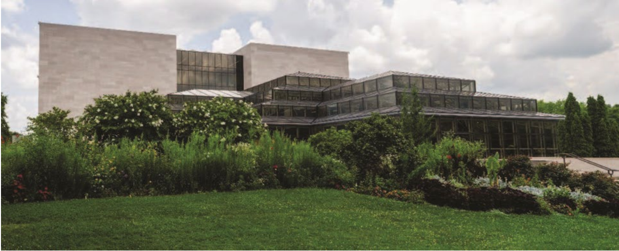
Restaurant addition and planted area at the east end of the NASM site. Historic American Building Survey, 2017.
