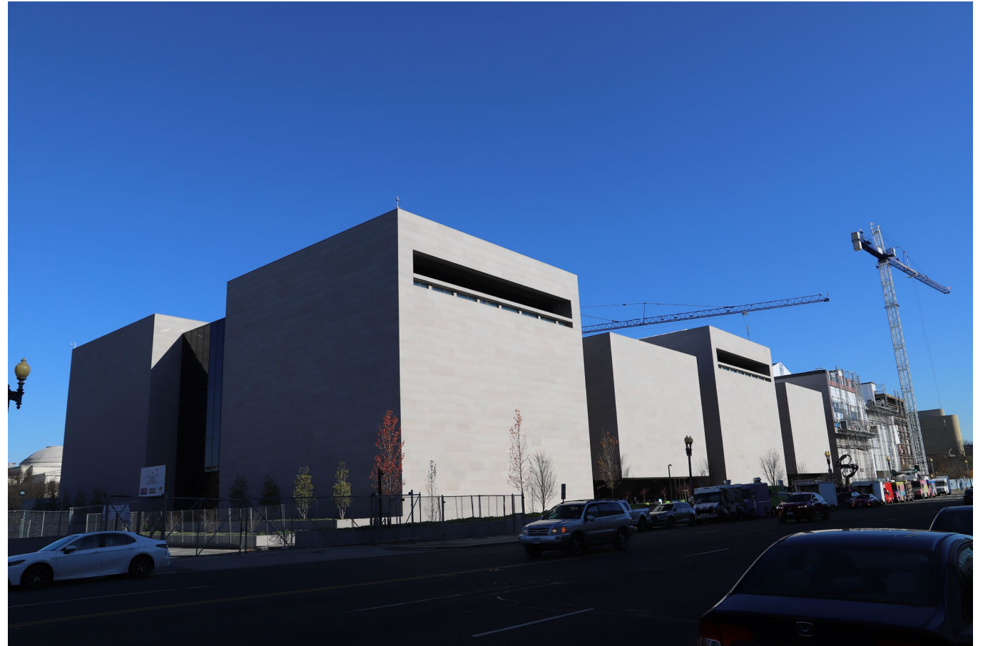
NASM viewed looking NE, November 2022.
