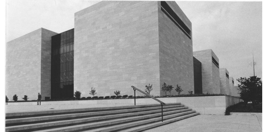
East Terrace, Looking South, c. 1976.
