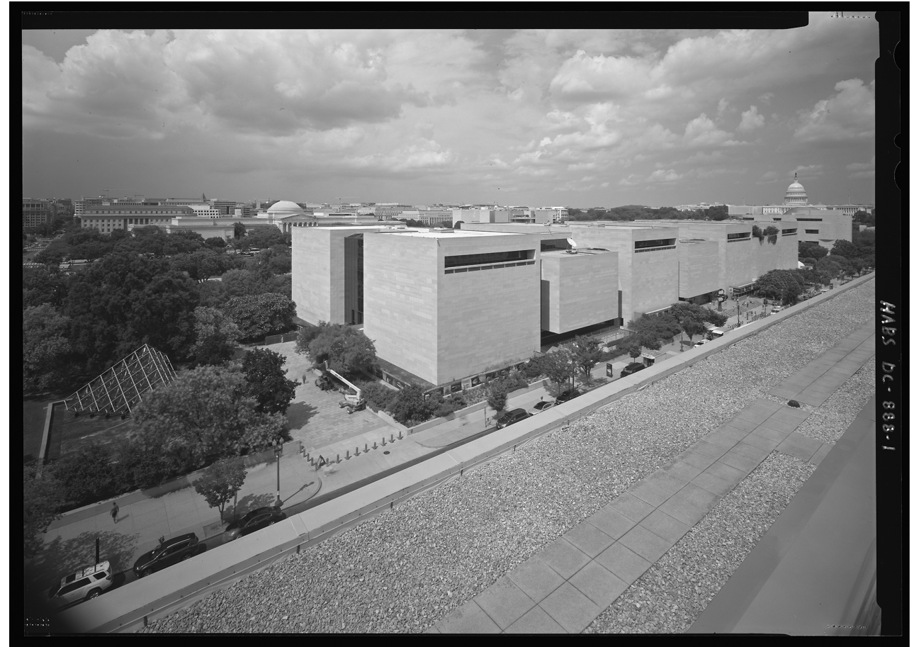
NASM Viewed Looking NE, Historic American Building Survey, 2017.
