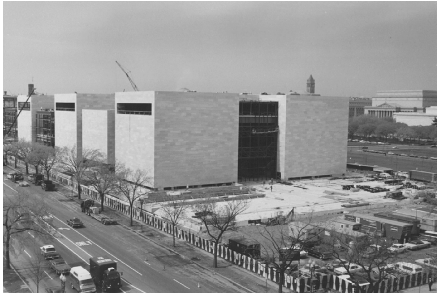
NASM and East Terrace Under Construction, 1974.
