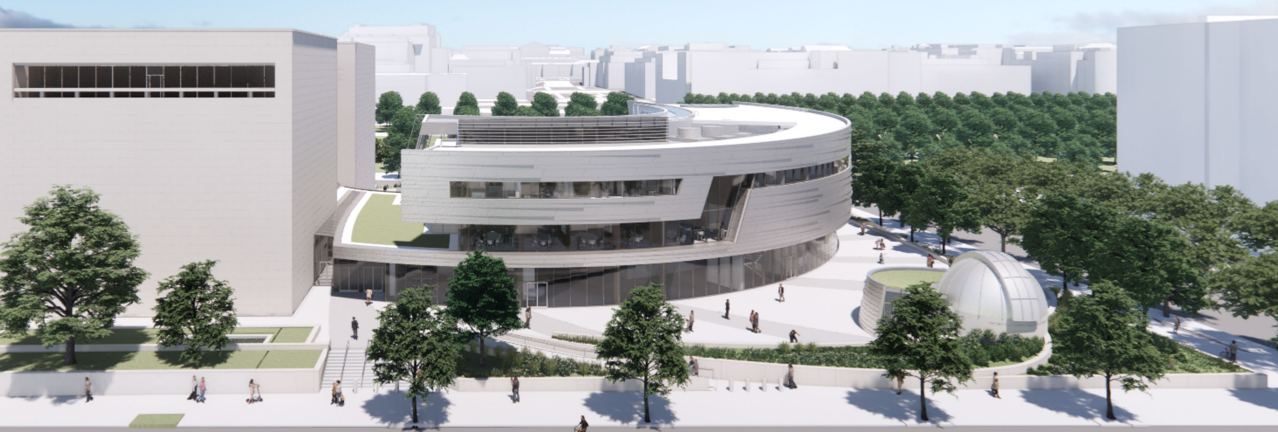
Construct Integrated Bezos Learning Center
