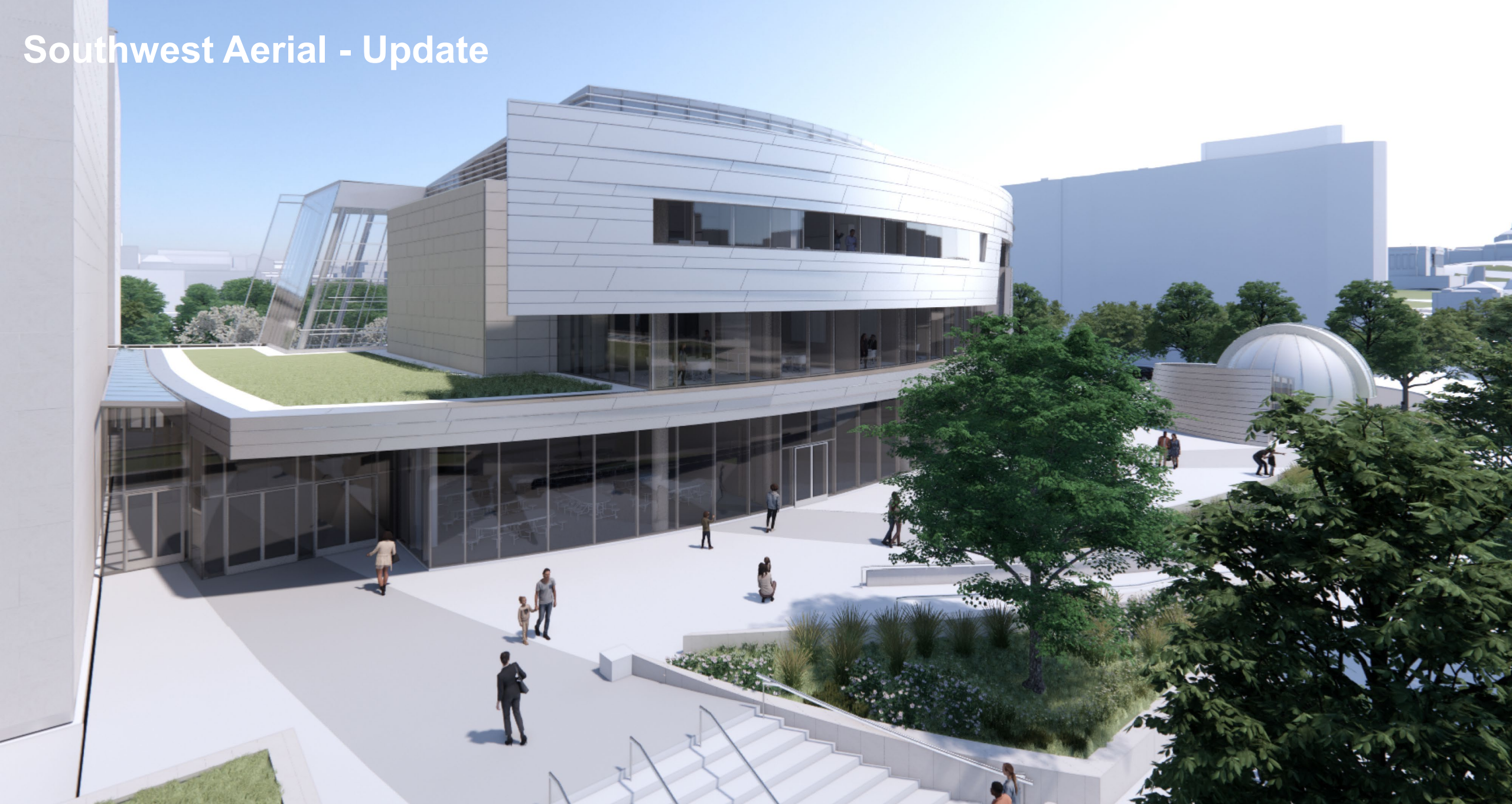
Construct Integrated Bezos Learning Center
