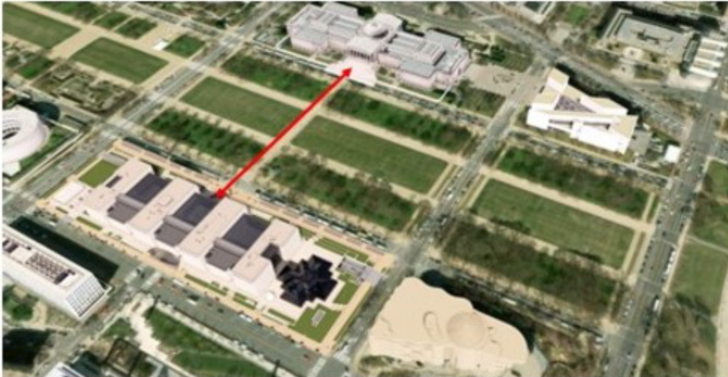
National Mall aerial view. Red arrow notes the 6 th Street axis and reciprocal relationship between the National Gallery portico and the NASM center glass atrium gallery.
