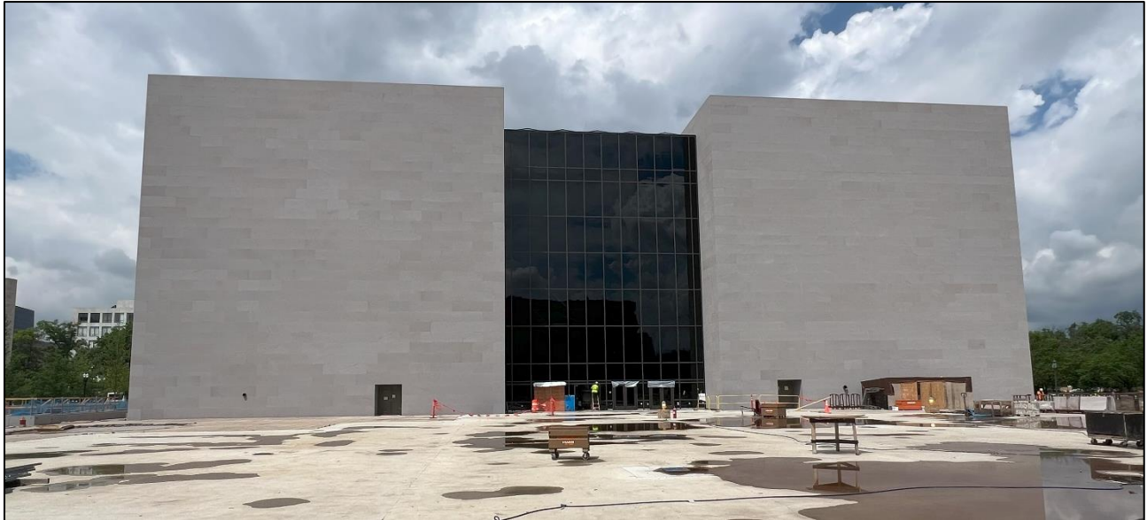
Extant view of NASM's east elevation, looking west, with the solid-void pattern, new glazing, and Colonial Rose Granite panels. (EHT Traceries, 2024)
