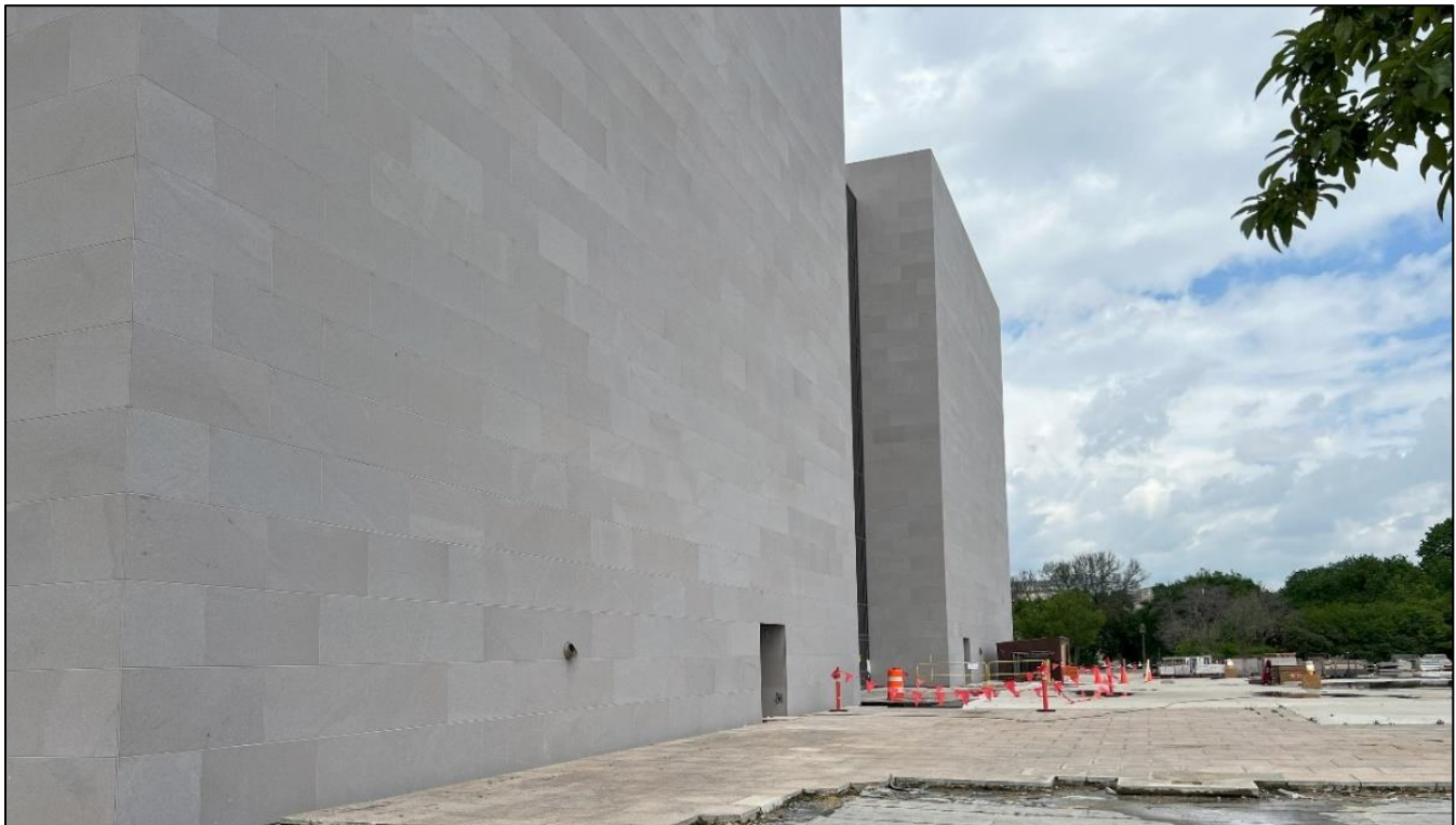
Southeast corner where the new connection will be made with the newly installed Colonial Rose Granite panels. (EHT Traceries, 2024)
