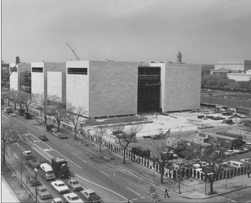
FIGURE 2: NASM AND EAST TERRACE, DURING CONSTRUCTION (1974)
