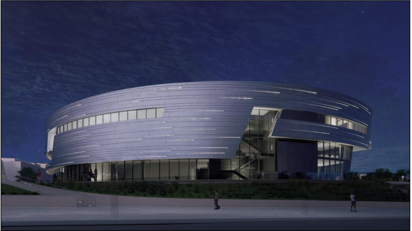
East elevation rendering at night of BLC and Hass Observatory with the integrated façade lighting within the metal panels. (Perkins&Will, 2024)
